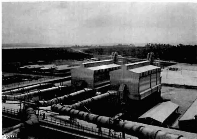
FIGURE 3. The system installed at Tucuru
