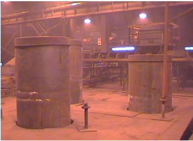
Figure 23. Electrode casing column paste covers all in place.
