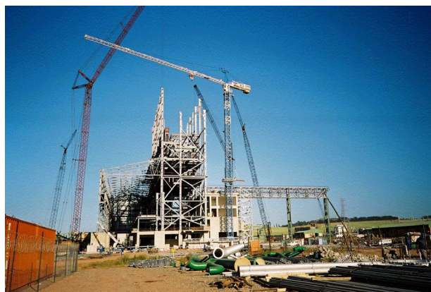
Figure 10. Ilmenite smelting plant under construction.
