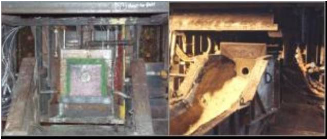
Figure 15. Water cooled tap hole.
