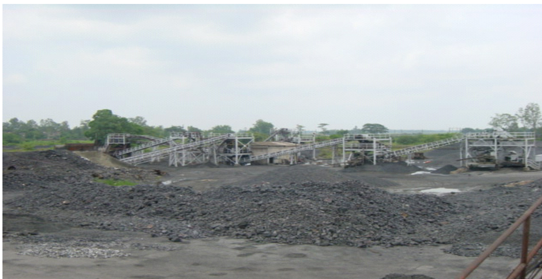
Figure 12: Metal Recovery Plant
