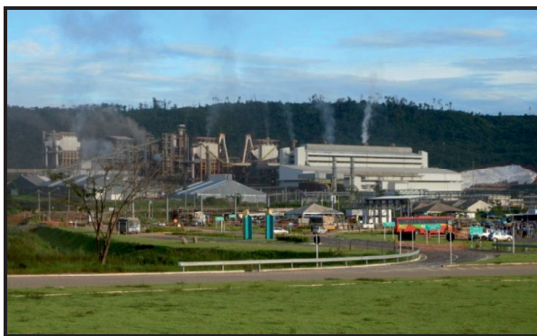
Figure : Vale Onça Puma Ferronickel Plant Brasil
