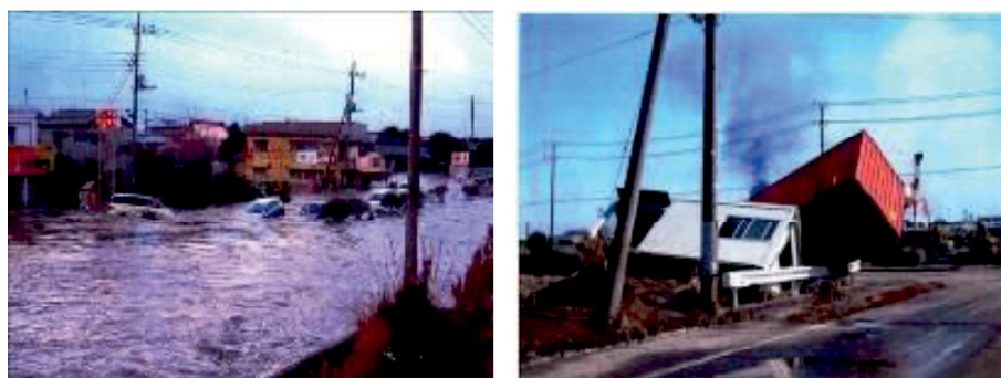
Figure 3.1.3: Tsunami damage near Kashima Port
