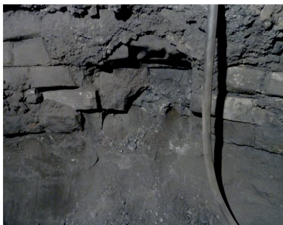
Figure 5: Condition of the Tapholes after four years of Operation
