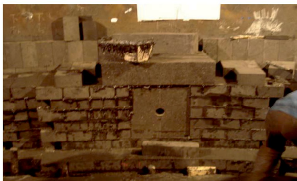
Figure 3: F101 Taphole under construction showing lintels in position
