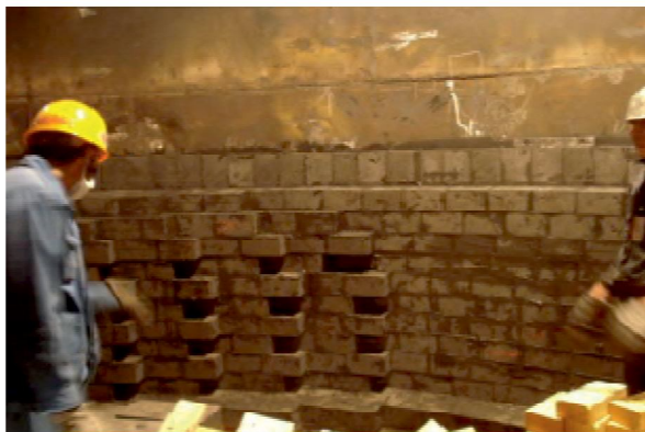
Figure 2: F101 Installation of HotPressed™ carbon bricks
