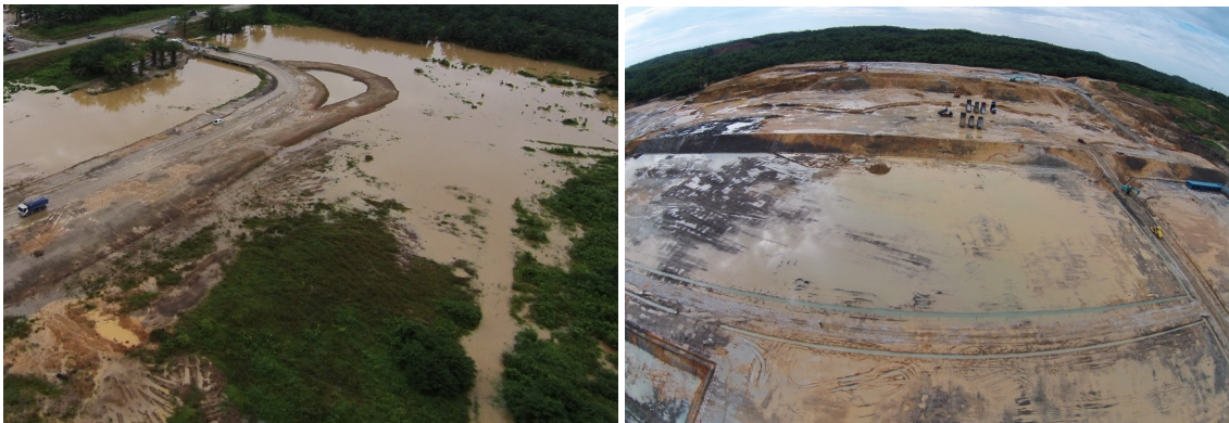
Figure 9: The construction site under water during the early works phase and terrace formation
