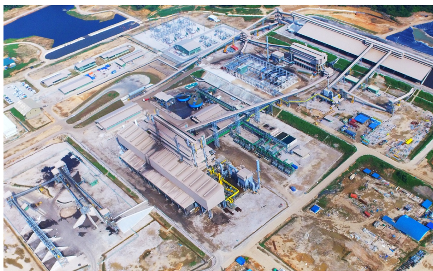
Figure 4: Aerial photograph of the Sakura plant after successful commissioning of F1 in 2016
