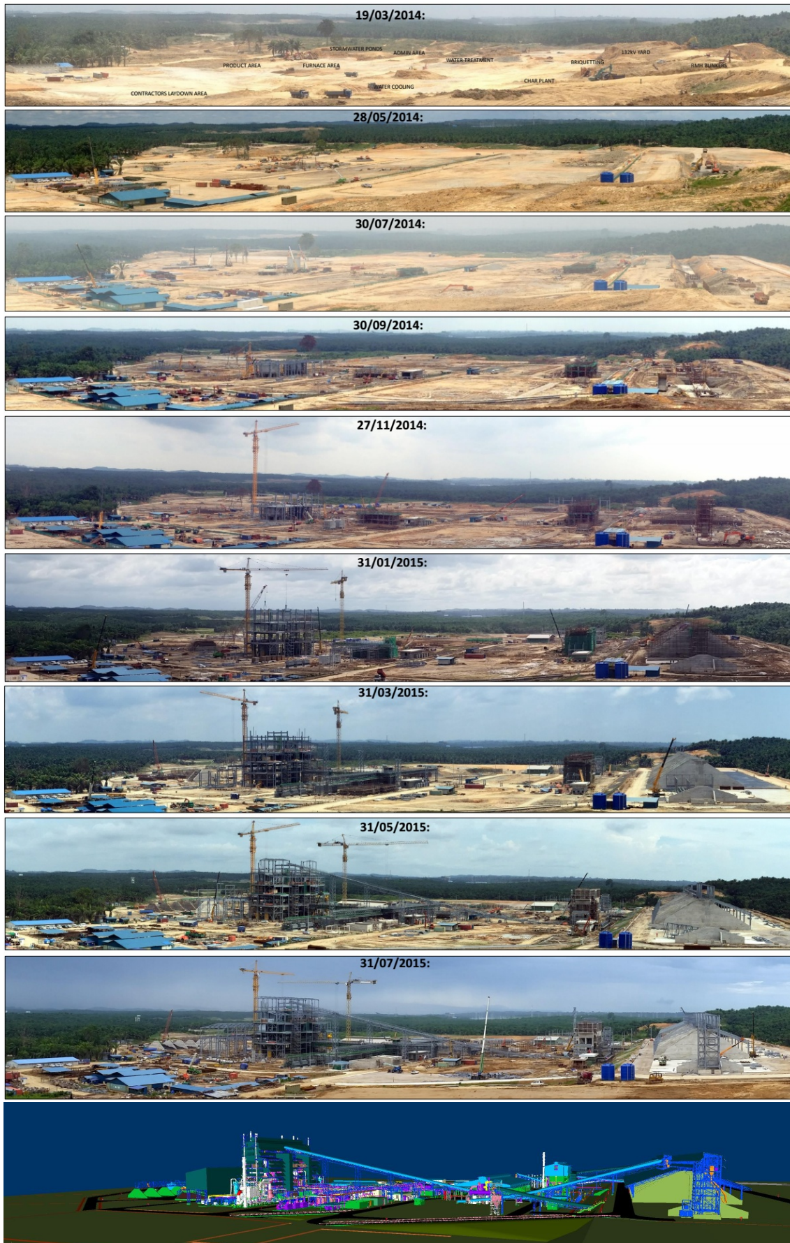
Figure 10: A photo trail showing the development of construction to realise targeted design
