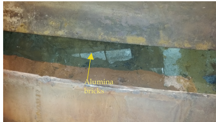
Figure 15: Brick removal from Furnace 1
